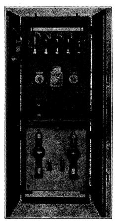
Fig. 9.—Front view of control panel for electrone tube, spot and line welder (Courtesy General Electric Co.)
