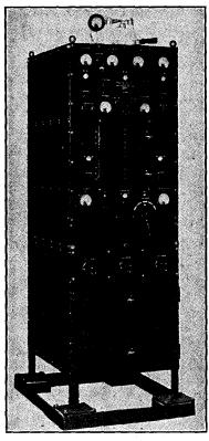
FIG. 4—This transmitter operates in the marine wavelength bands between 375 and 500 kilocycles (600-800 meters) and 5,500 to 17,000 kilocycles (17-54 meters). The band from 375 to 500 kilocycles is the one generally
